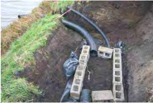
Two types of otter holt in construction. Left, an underground one built into the side of a drain that will be covered and restored to its original profile and right, an above ground one that is being covered by logs from the adjacent coppiced willow.
