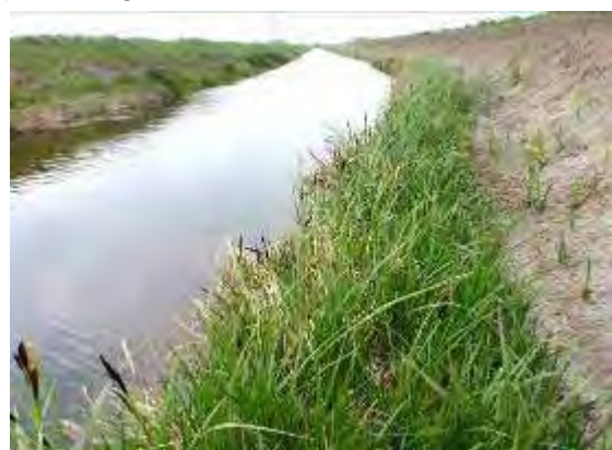
Left, a band of sedge protects the margin of a March Third DDC ditch and right, on the same ditch the sedge has been retained as a stabilizing ledge and a valuable habitat for water voles and other wildlife when the bank was re-profiled.
