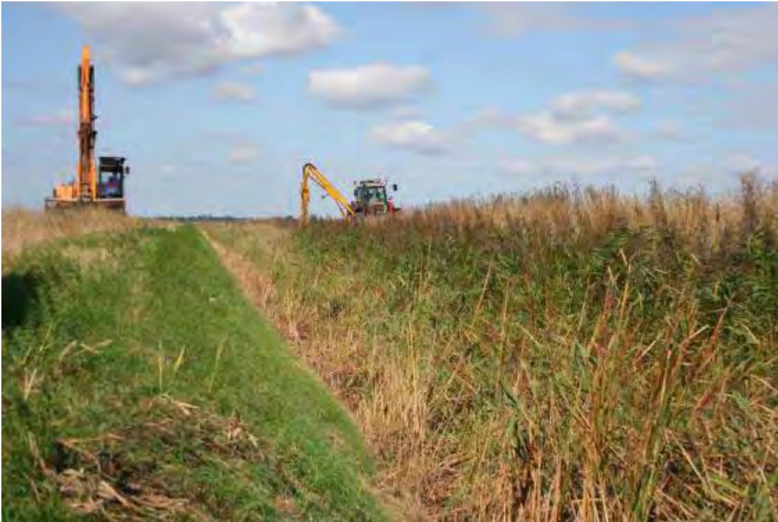
A well maintained sward retains bank stability. Wimblington Combined IDB.
