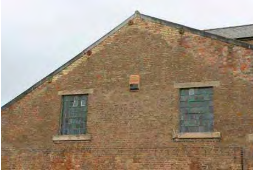
A bat box sited high on the gable end of Mepal Pumping Station, Sutton & Mepal IDB
