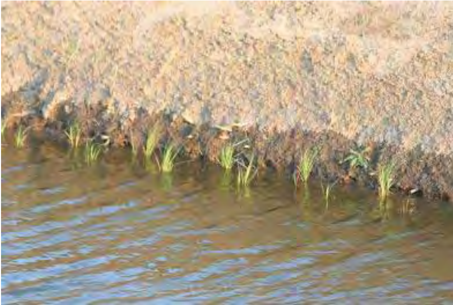
Sedge plugs planted at the toe of a newly profiled drain bank in March & Whittlesey IDB that will form a protective margin in due course.
