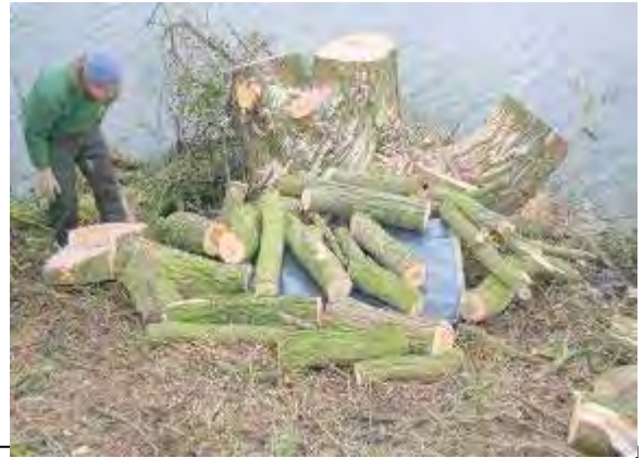
Two types of otter holt in construction. Left, an underground one built into the side of a drain that will be covered and restored to its original profile and right, an above ground one that is being covered by logs from the adjacent coppiced willow.
