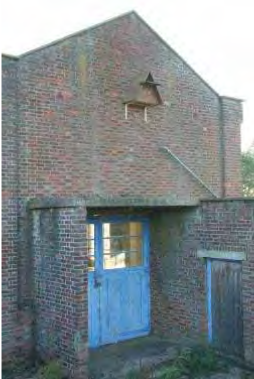
An external barn owl box sited on a former pumping station building at Glenhouse in Manea and Welney DDC District.
