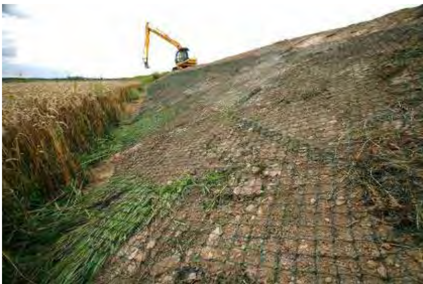
To prevent badgers returning to the site, chain link fencing is pinned to a newly reconstructed bank on the Black Ham following sett collapse under licence. It will be covered by a thin layer of soil.
